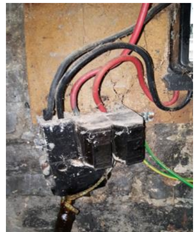
Examples of a cut-out that is clearly not securely fixed onto a wall
