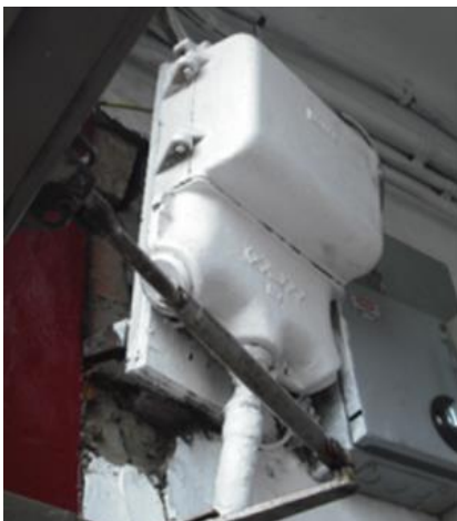
Examples of a cut-out that is clearly not securely fixed onto a wall
